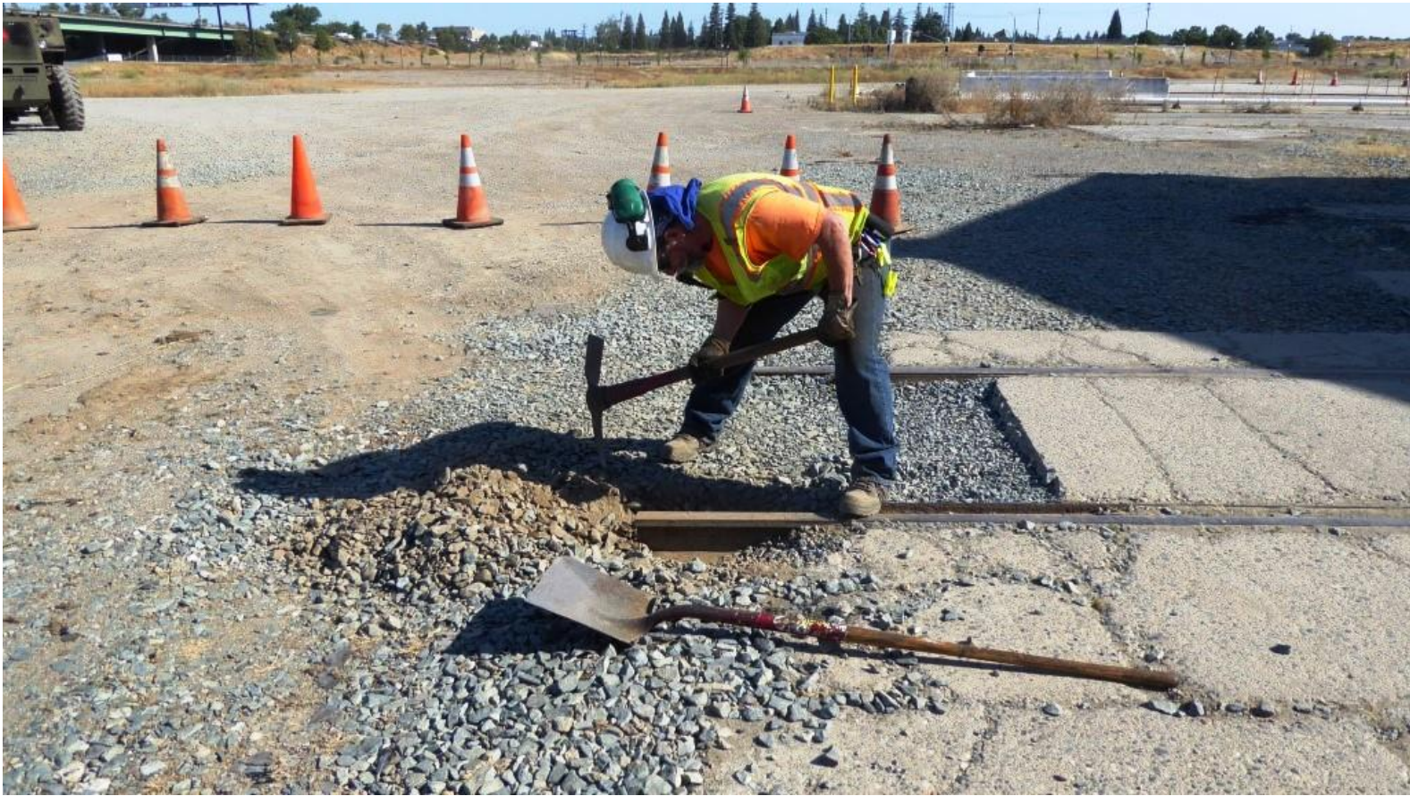
Joe digs out the ends of the Firing Line rails
