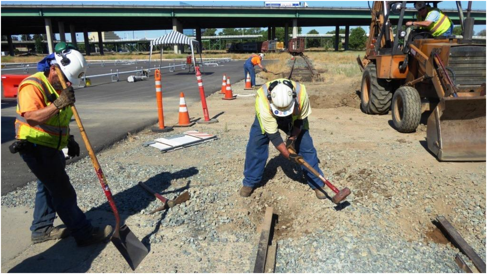
Mike pounds the rail with a sledgehammer to knock-off concrete embedded in the web
