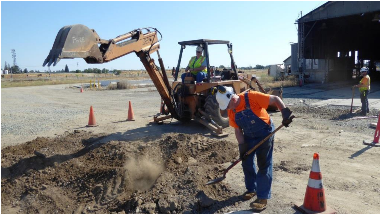
As Chris digs out the road-bed, Clem comes in to start cutting an edge
