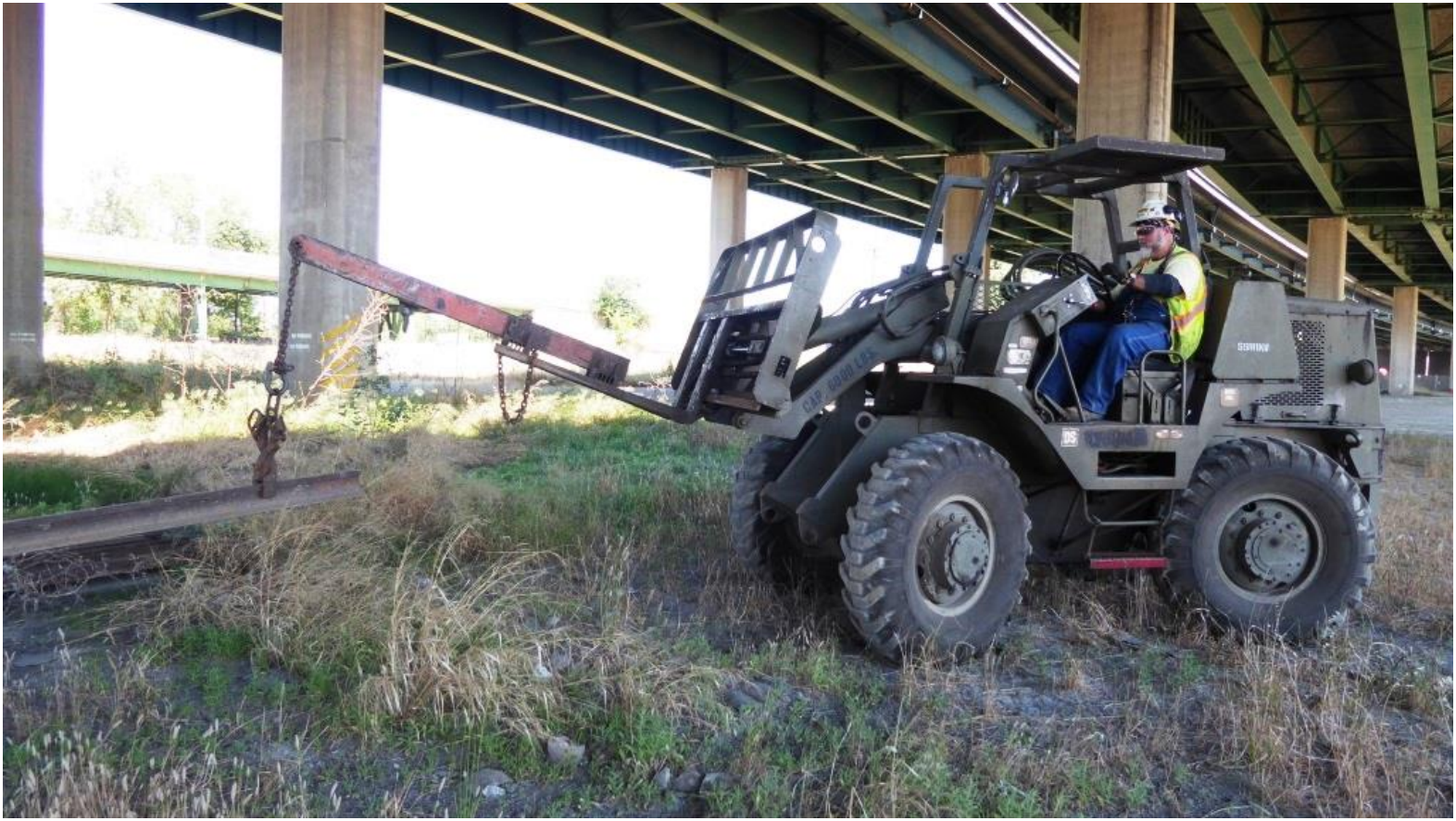
Mike grabs a stick of rail from our stockpile under the freeway...
