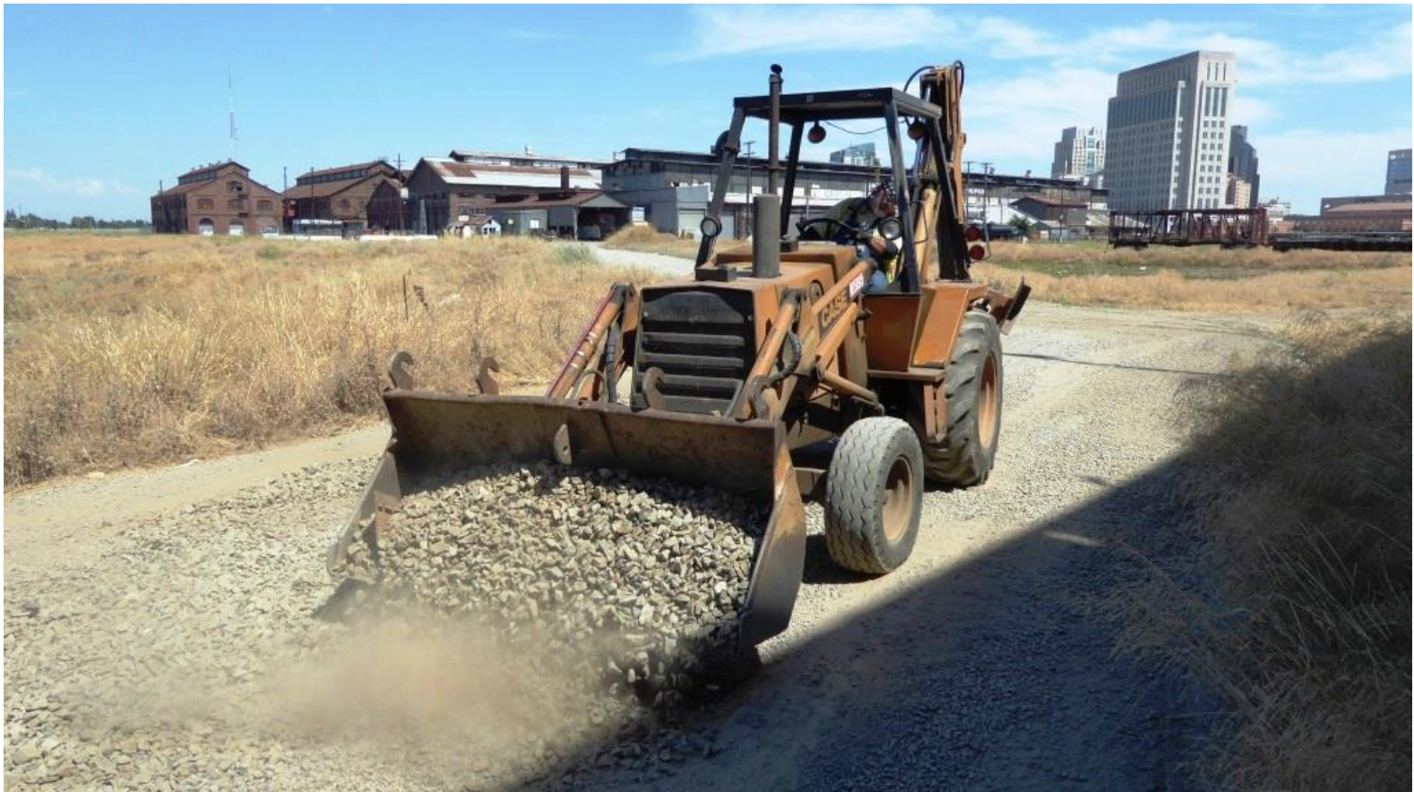
Mike on the back-hoe fills in road ruts with old rock and spoils from the job-site
