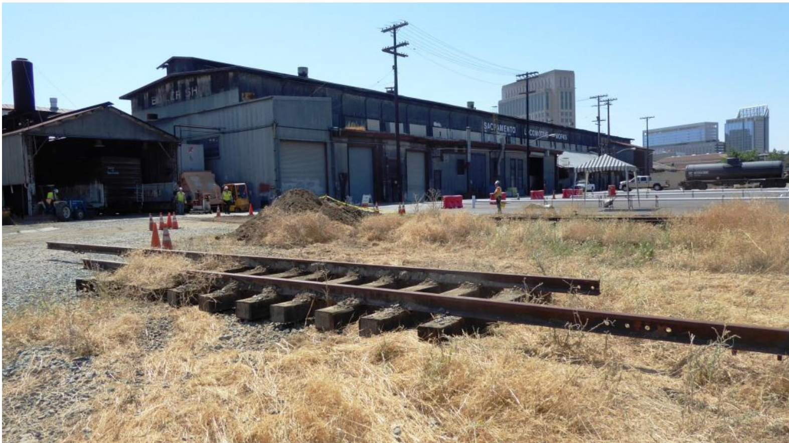
...And spots it in a position where it's ready to be installed
