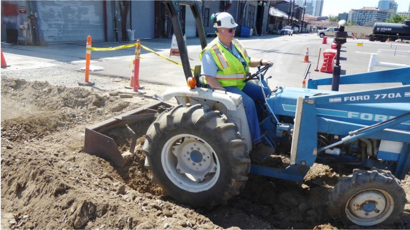
Chris uses the grading box on the tractor to move dirt
