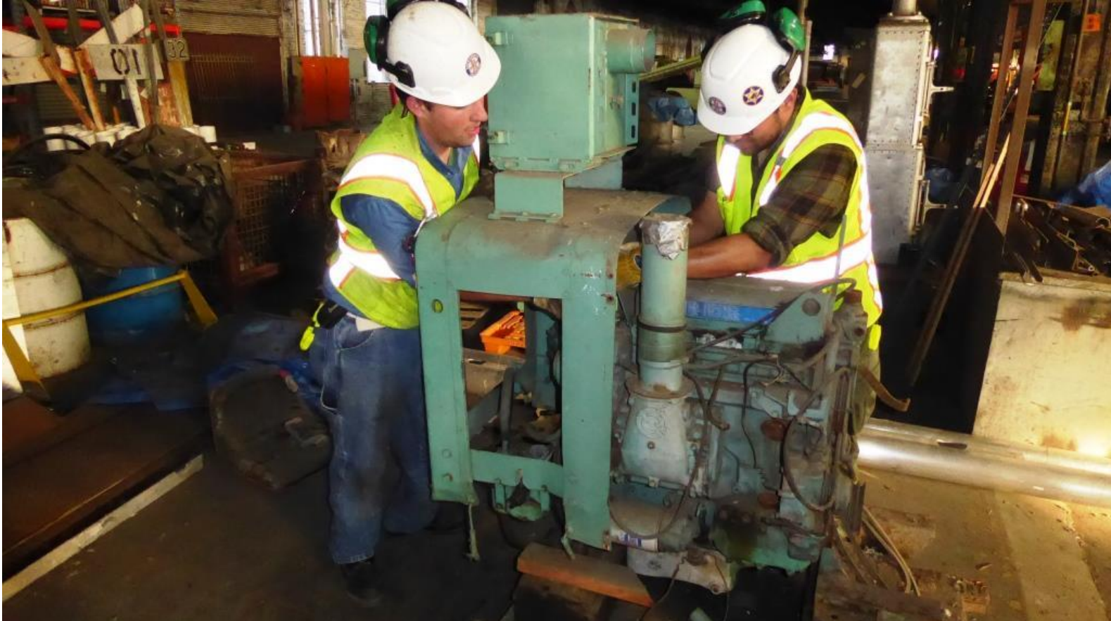
Weston and Kyle start dismantling the engine
