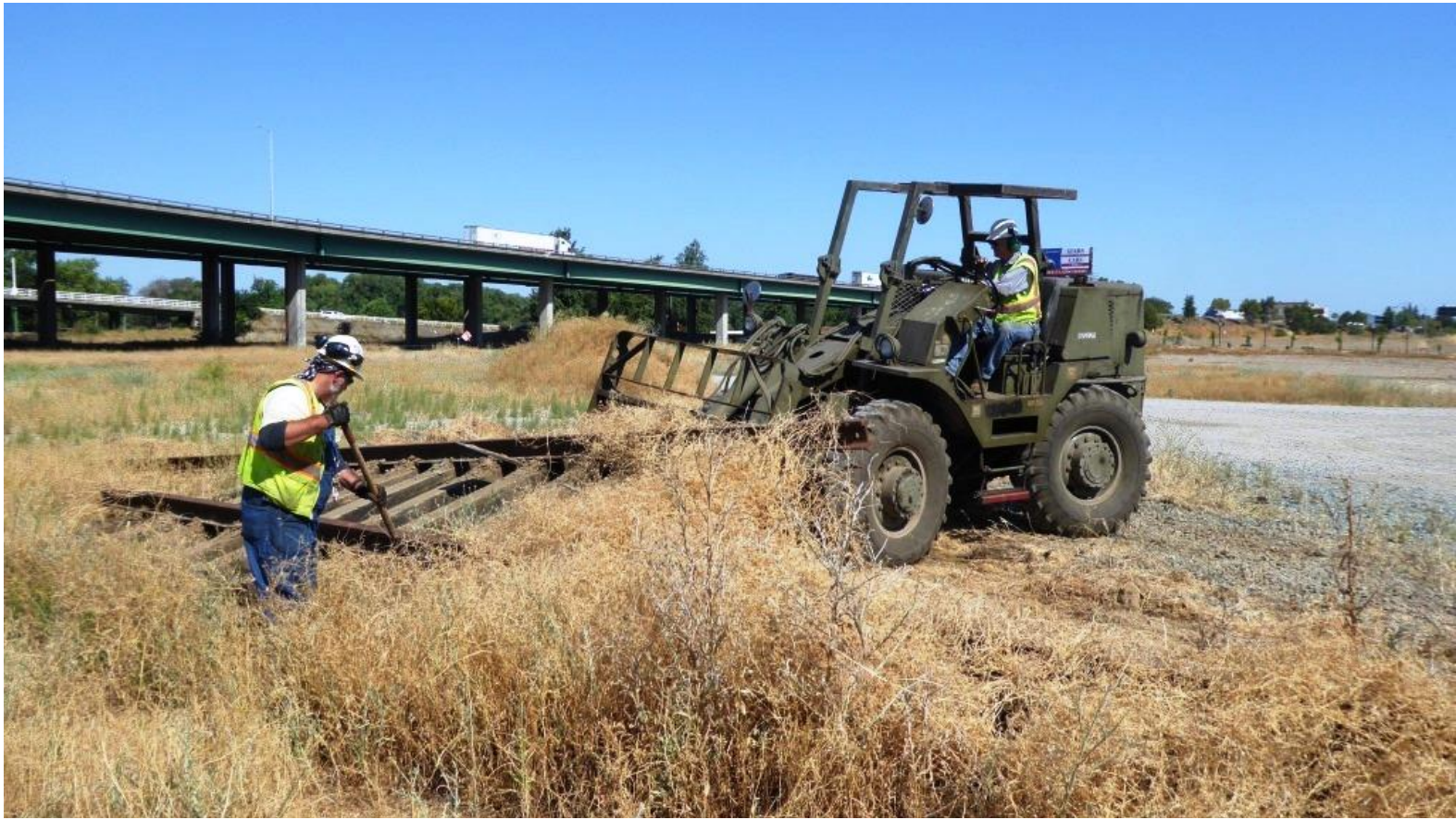
Steve grabs the panel of track with the forks of GM2...
