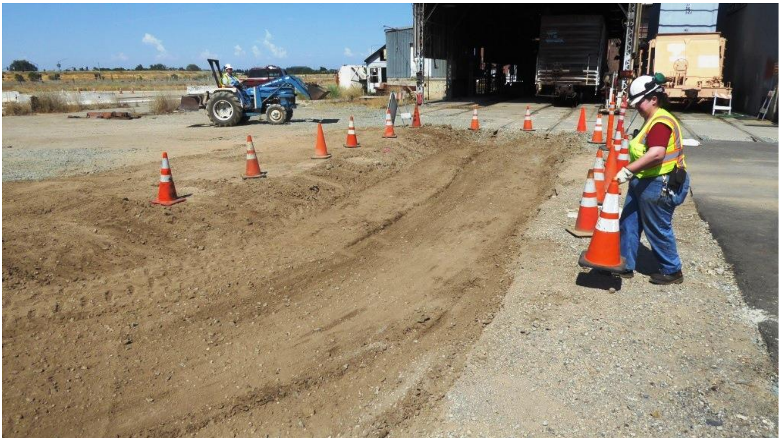
Heather sets up warning cones around the new track-bed – which is actually deeper than it looks in this photo
