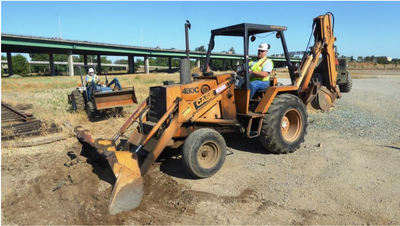
Chris deepens the hole with the back-hoe's bucket while Alan stands by on the blue tractor to haul the dirt away
