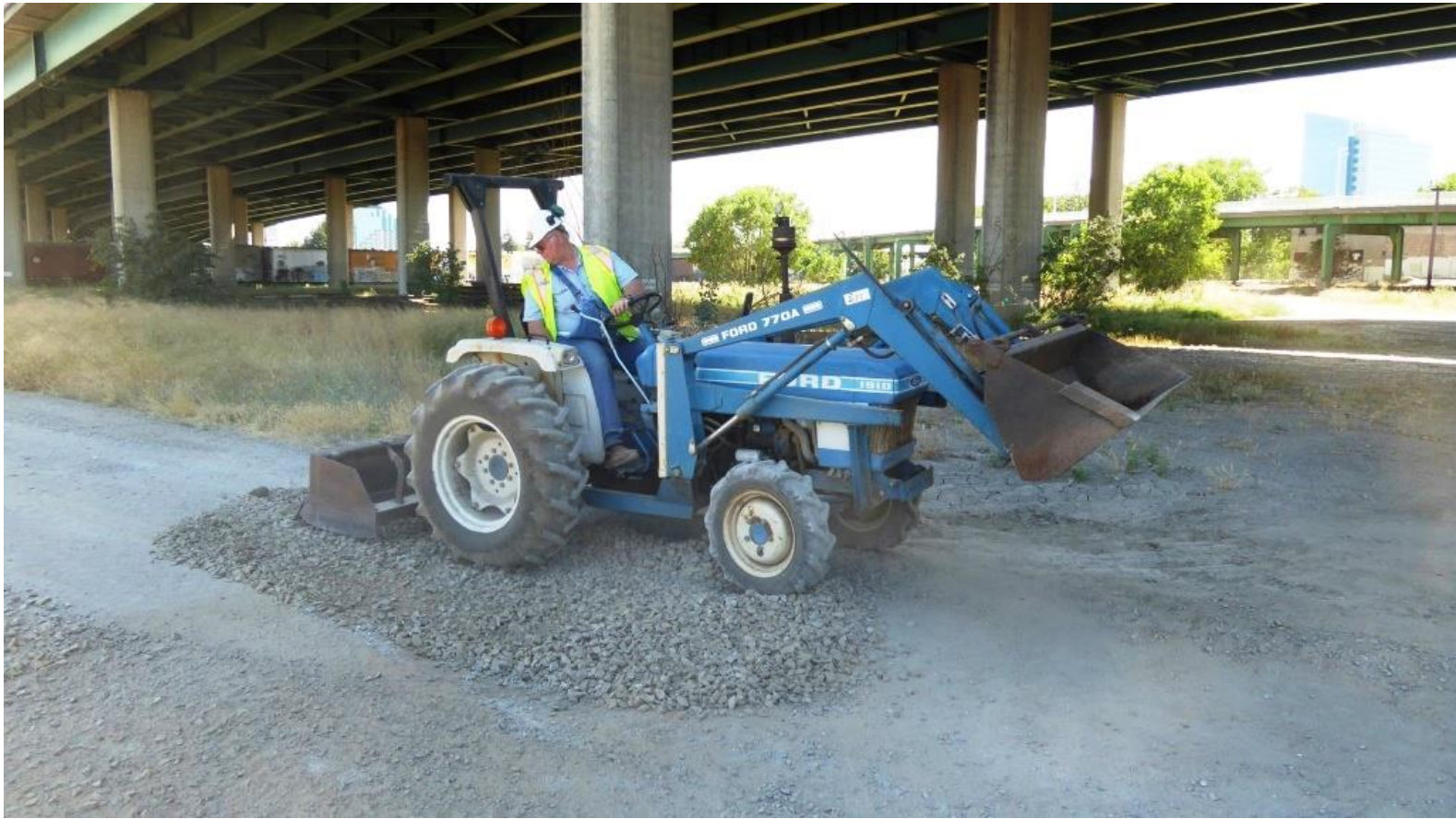
Chris on the blue-tractor uses the grading box to compact the rock and smooth the surface
