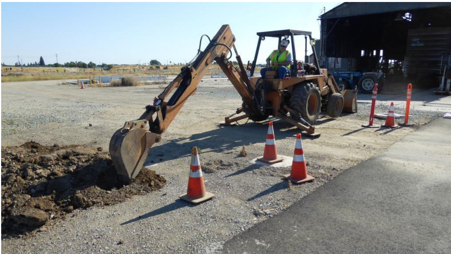
Let the digging begin! Chris uses the back-hoe to break-up the hard, compacted soil
